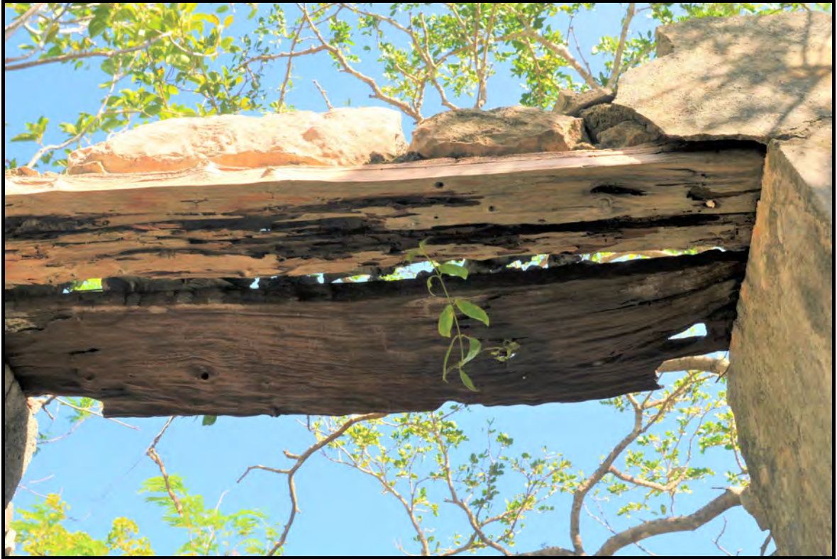
Plate 17a. Structure 6(a). Lignum vitae lintel over window opening.
