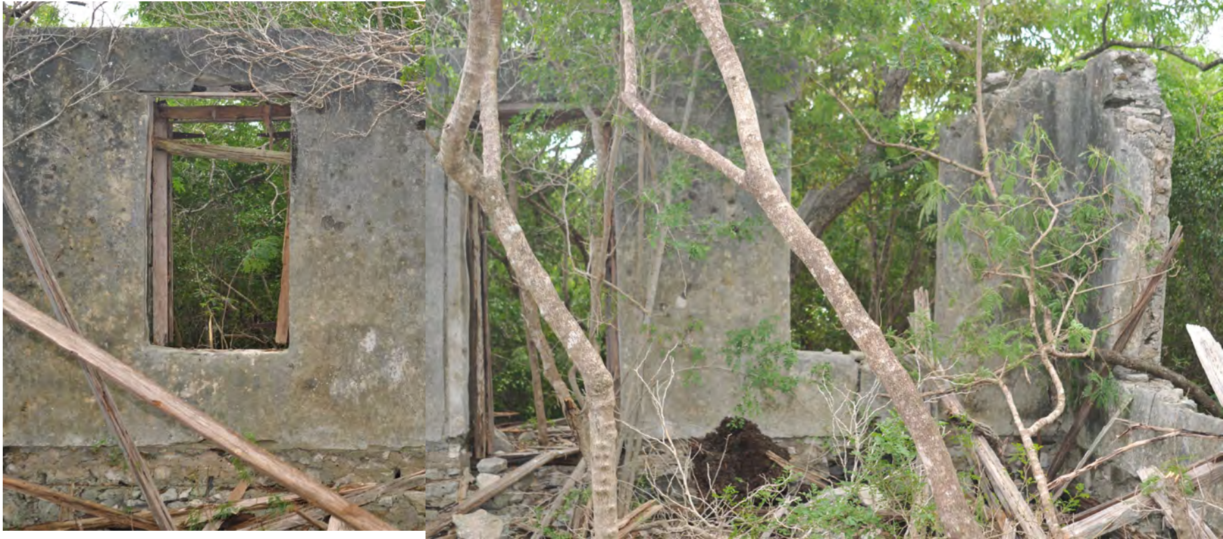
Plate 9. Structure 5. South facade, interior view (composite).
