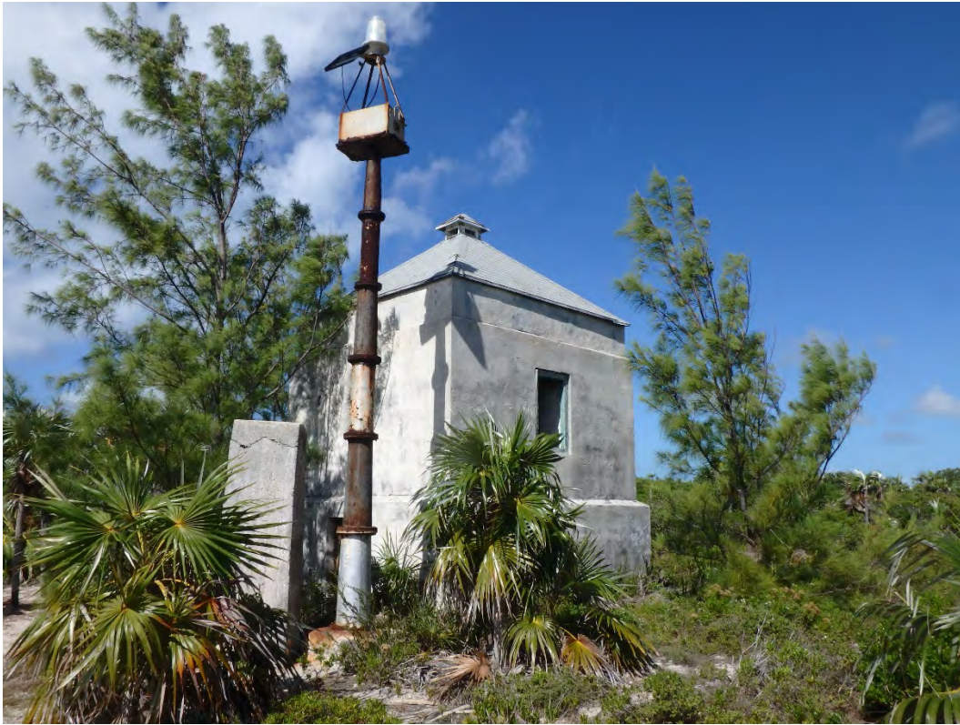
Existing Lighthouse Structures
