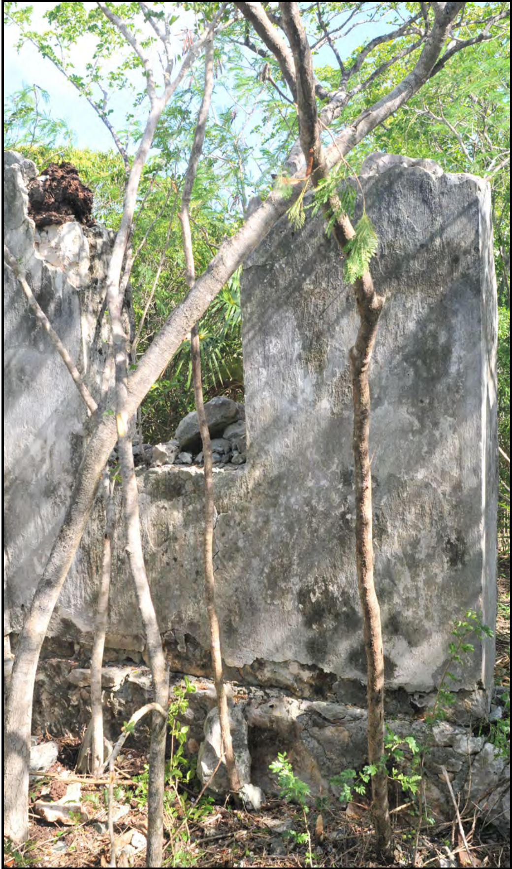
Plate 13. Structure 6(a). Detail of northeast exterior corner.
