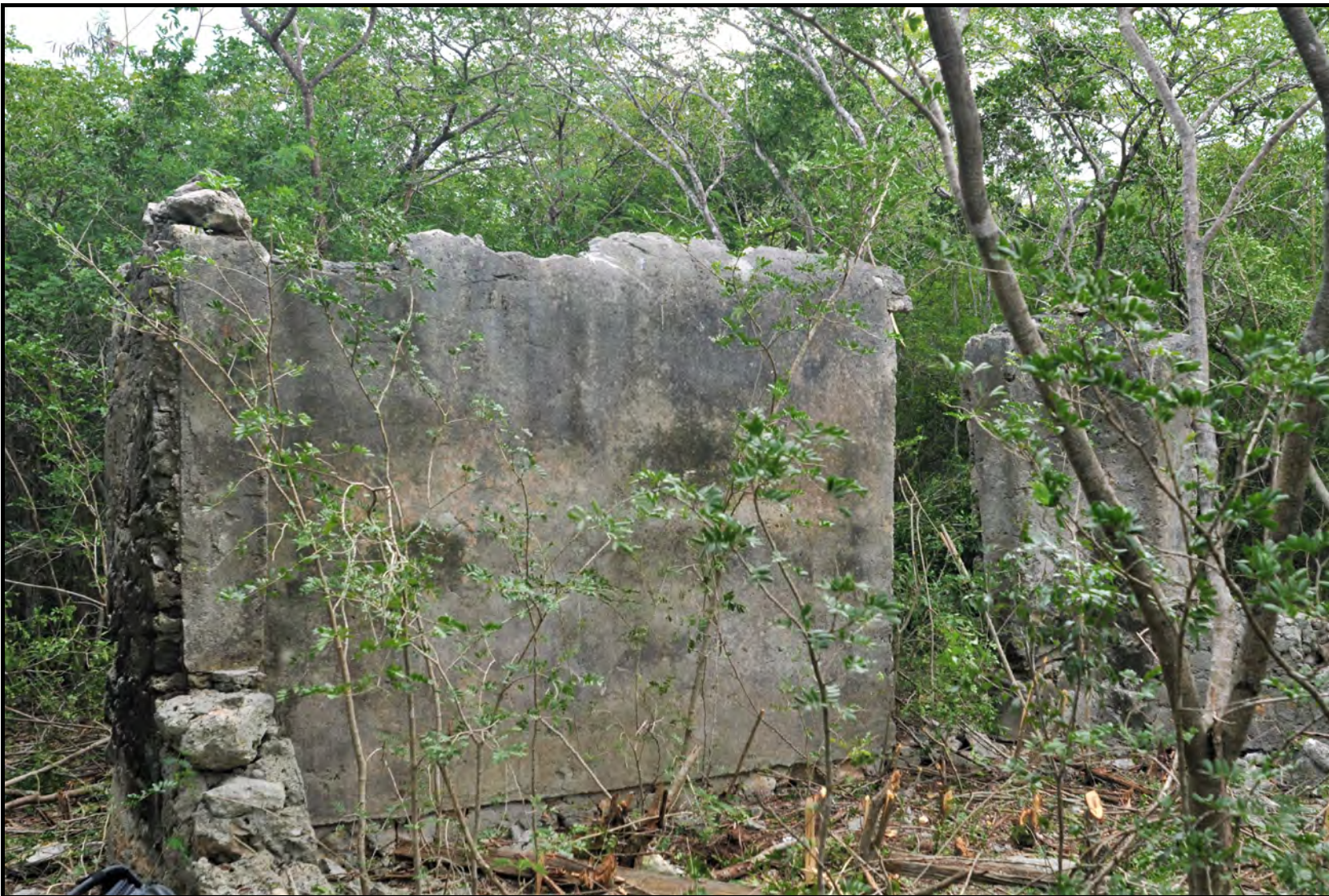
Plate 6. Structure 3. Oblique view, interior north facade.
