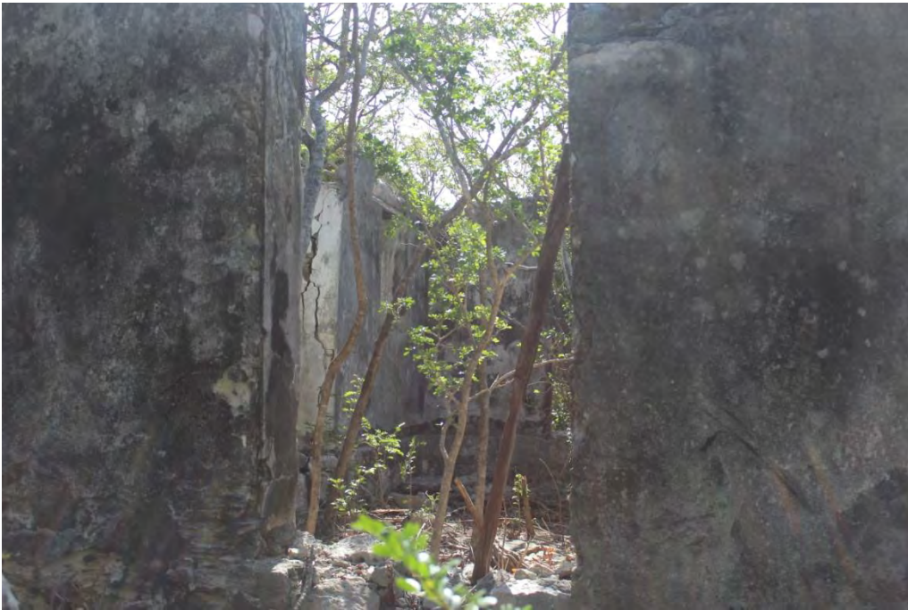
Fig.2 Structure 1 was constructed using relatively small cut limestone blocks.
