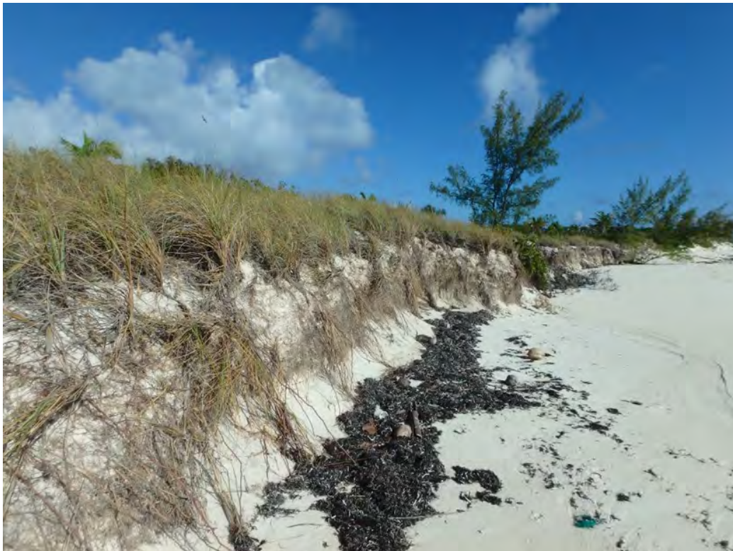
Photo 4-6. Area of Moderate Erosion
