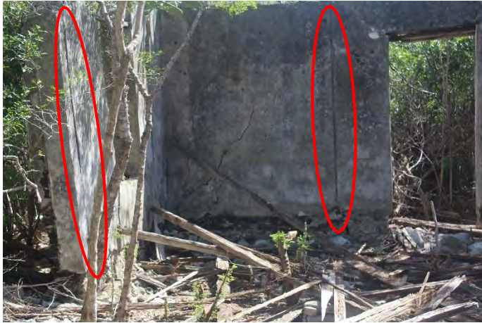
Fig.15a Lines in the stucco indicate original wooden dividing walls.
