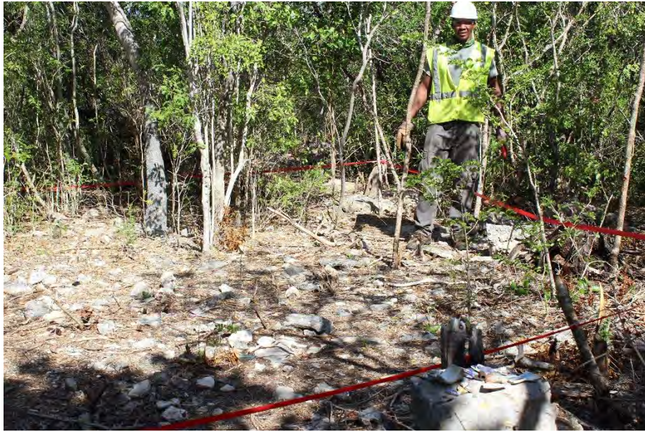
Fig.6 Red survey tape outlines wooden post holes cut into the bedrock for a wood-frame building.
