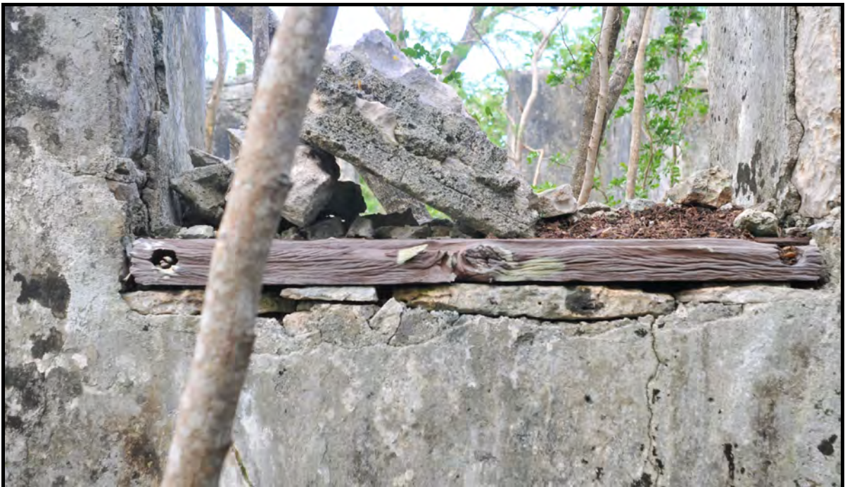
Plate 17b. Structure 6 (a). Lignum vitae window sill.
