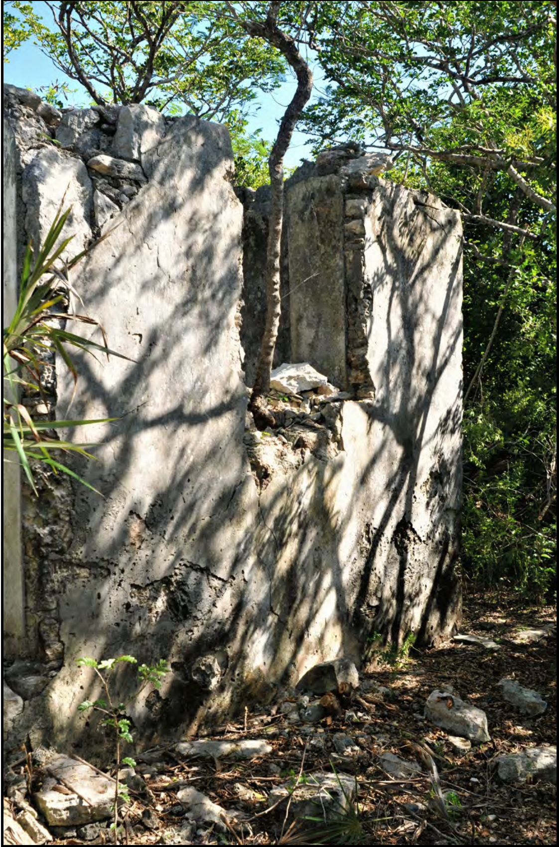
Plate 14. Structure 6(a). Detail southwest exterior corner.
