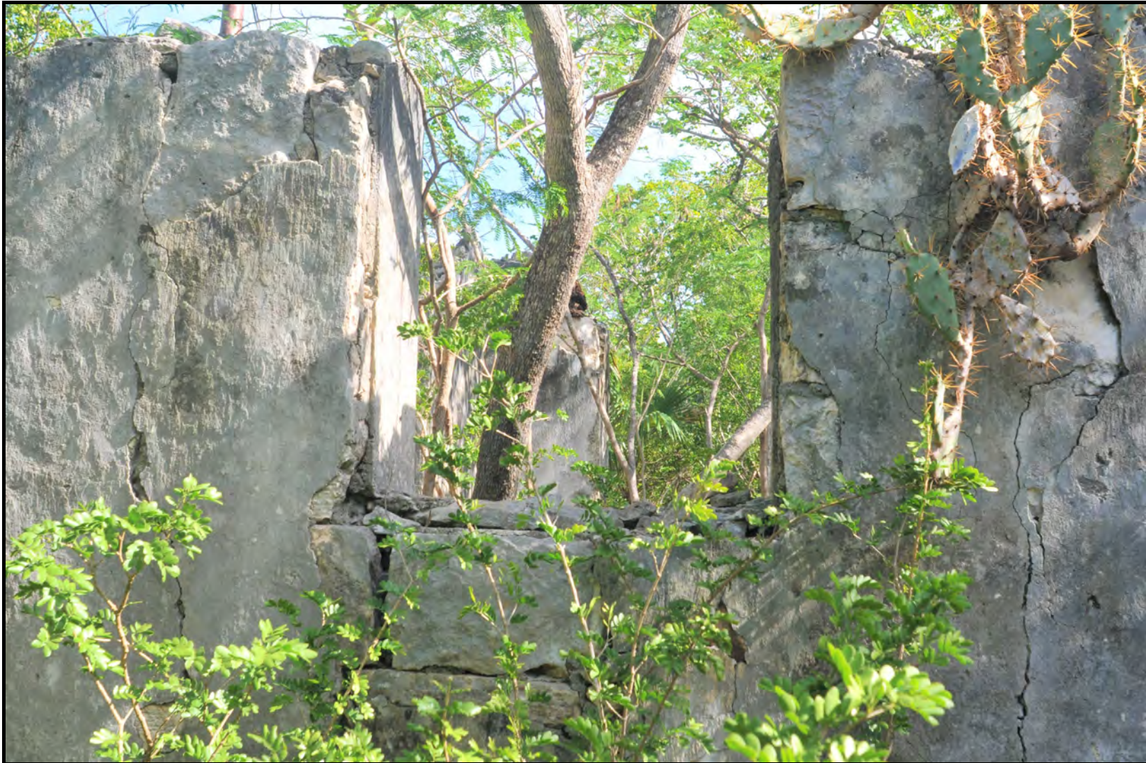
Plate 15. Structure 6 (a). Detail of west facade showing cut stone masonry around window opening.
