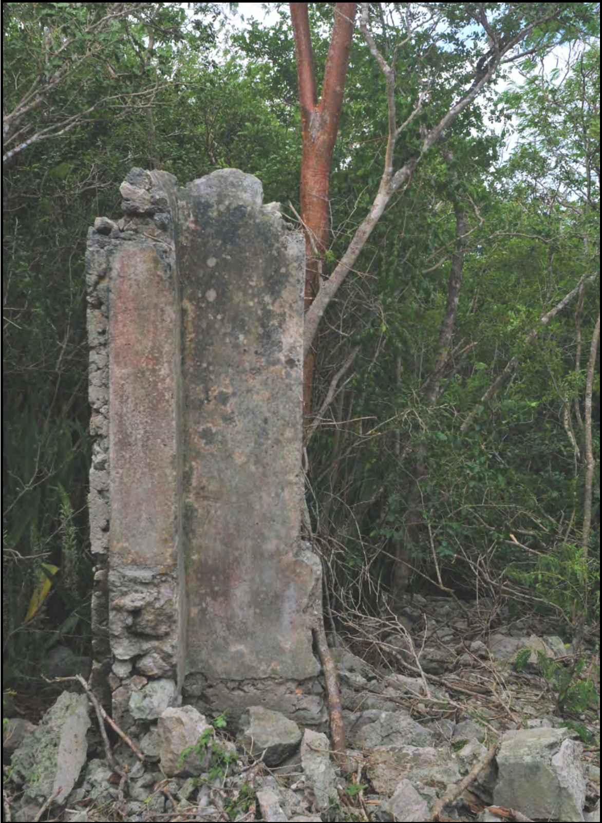
Plate 5. Structure 3. Remnants of southeast exterior corner showing traces of windows.
