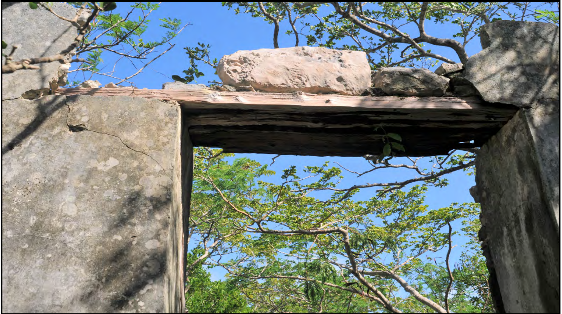
Plate 18. Structure 6(a). East facade, detail of lignum vitae lintel over window opening, interior view showing bearing.
