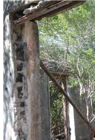
Fig.15b Wire nails secure hand-planed wooden door and window frames.
