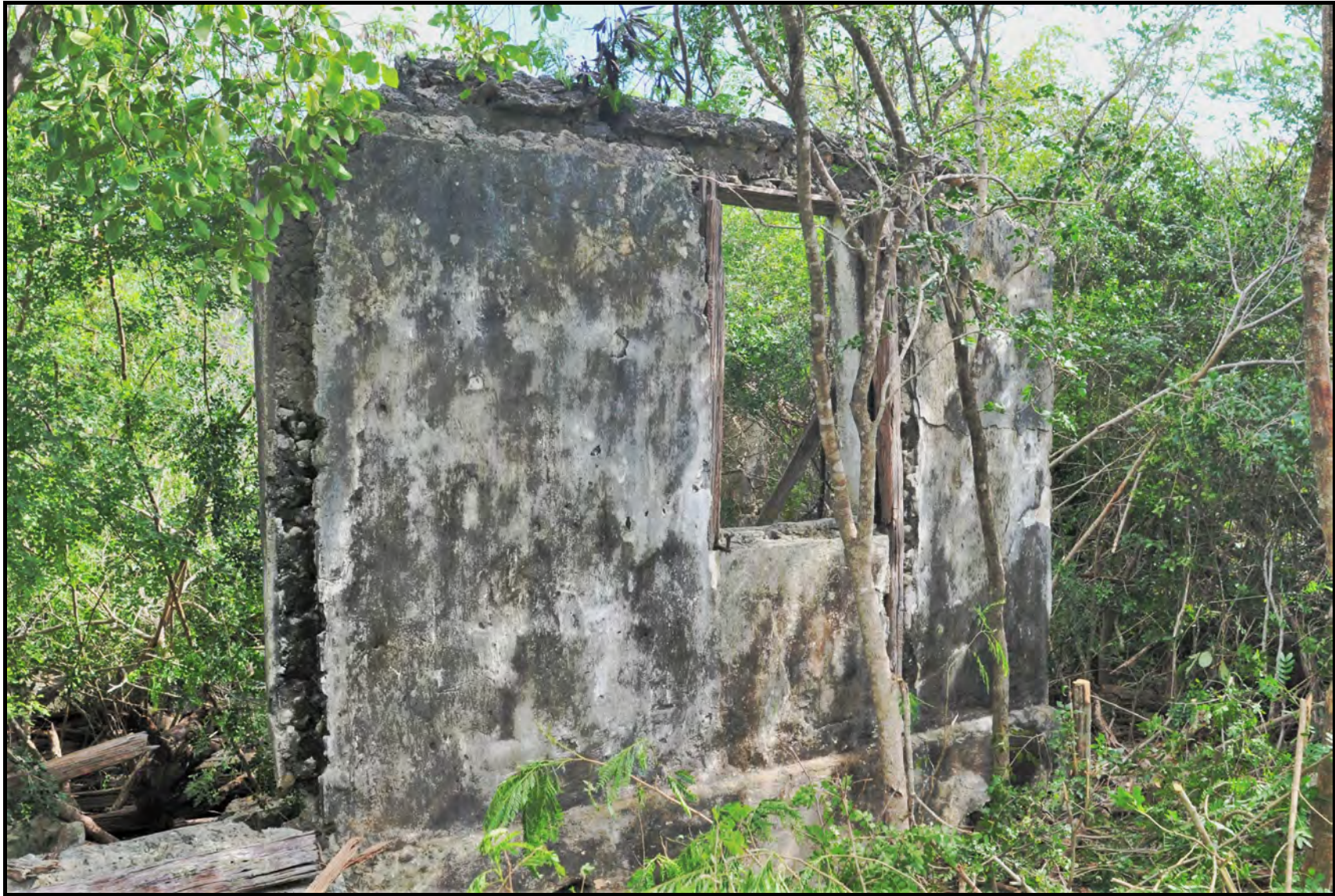
Plate 1. Structure 1, detail of west facade showing doorway and window opening.
