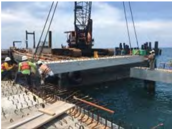
Photo 5.3-5: Setting Deck Planks
