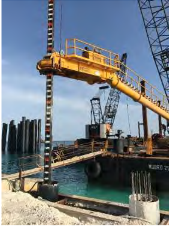
Photo 5.3-1: Crane-Mounted Hain's Drill for drilling rock sockets below pile tip elevation.
