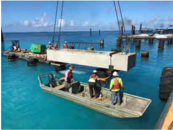
Photo 5.3-4: Setting Pre-Cast Cap on Piles
