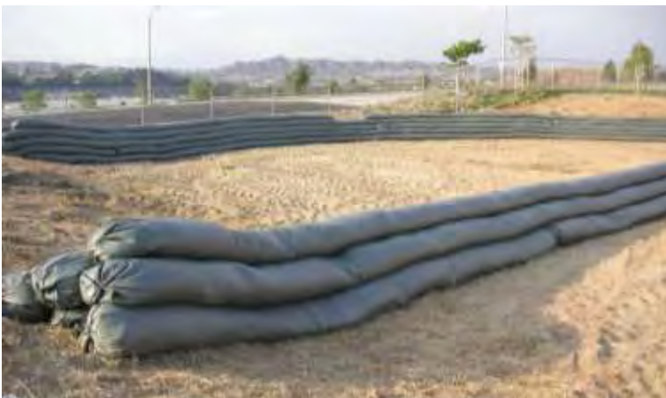
Photo 4: Gravel Bag Berms
