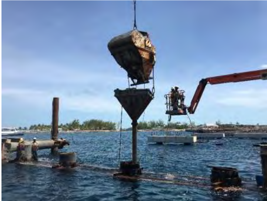
Photo 5.3-3: Tremie pipe with hopper being used to place concrete.
