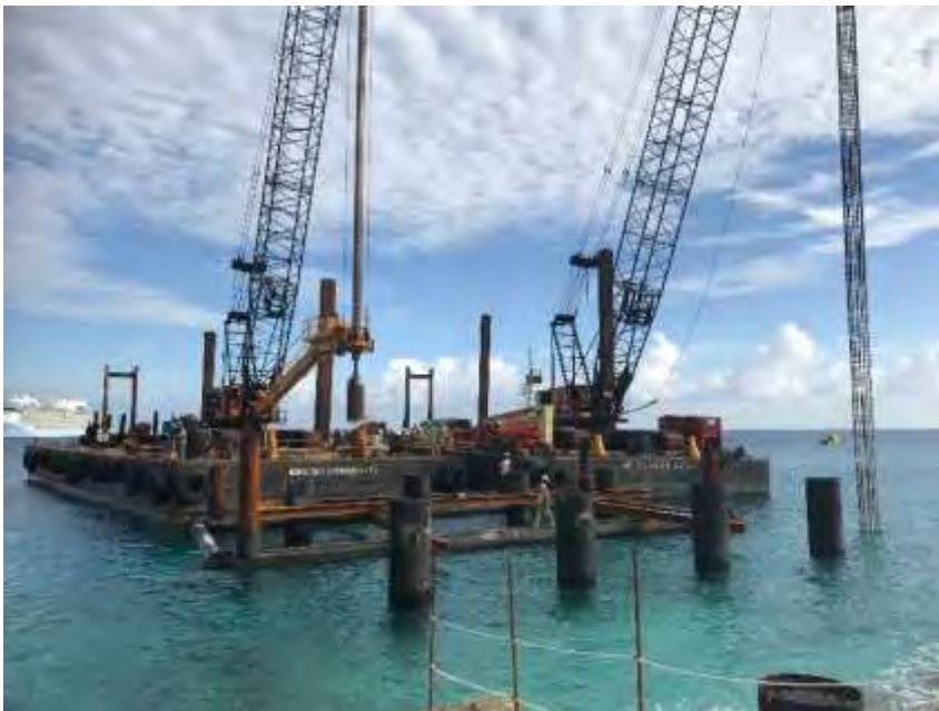
Photo 5.3-2: Final Clean-out of Pile and Rebar Cage Installation
